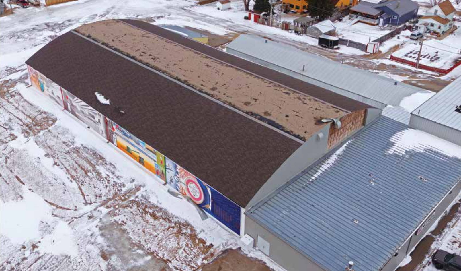
The skating rink in Avonlea also suffered significant shingle loss to its roof. Photo by Allan Spriggs Drone Photography & Video.
